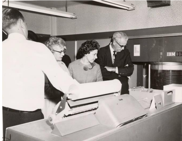
IBM 305, Random Access Memory Accounting, the first hard disk drive system, developed in 1956, offering ability for real-time accounting. Real-time was both a challenge and opportunity for COBOL programmed systems that tended to be batch/remote batch. (Image: Charles Babbage Institute Archives)
